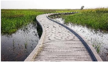
Boardwalk through a Stormwater Management Area
