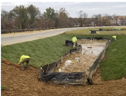
Converting a Former Sediment Retention Pond
