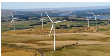
Manhinerangi Wind Farm
