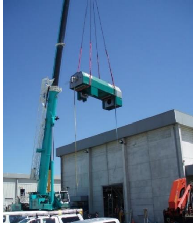
Mangere WWTP, Centrifuge and Conveyor Upgrades, Watercare Services
