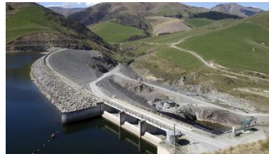
Opuha Dam, South Canterbury
