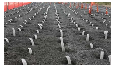
PJK Expressway, Wick Drains
