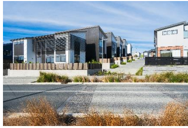
Raingardens in a New Housing Area
