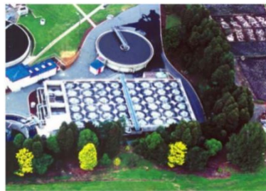
Tokoroa STP, South Waikato District Council
