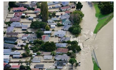
Edgumbe, Stopbank Failure
