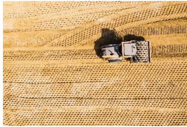
Large-scale Subdivision Earthworks
