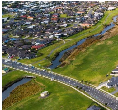
Low Flow Channel within a Managed Floodplain
