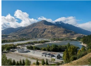
Project Shotover WWTP, Queenstown Lakes District Council
