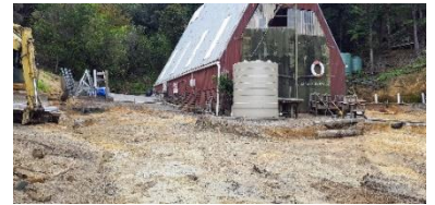
Boat Yard Remediation Validation, Opua
