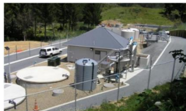
Kawakawa Bay WWTP, Watercare Services Ltd
