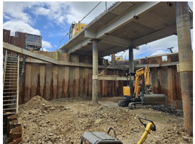
Te Kowhai tidal gate, construction below river level
