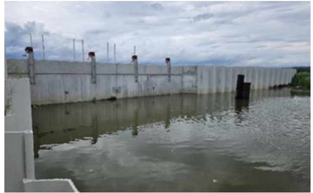
Te Kowhai Tidal Gate Project - Design & Construction
