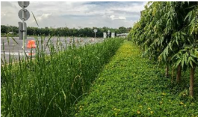
Grassed Swale Drain
