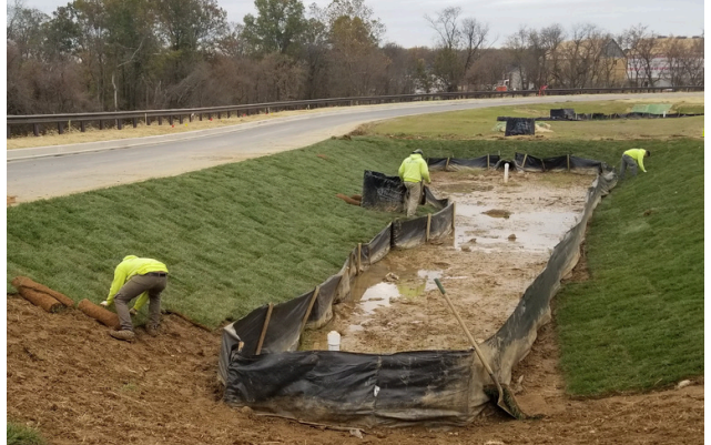
Converting a Former Sediment Retention Pond
