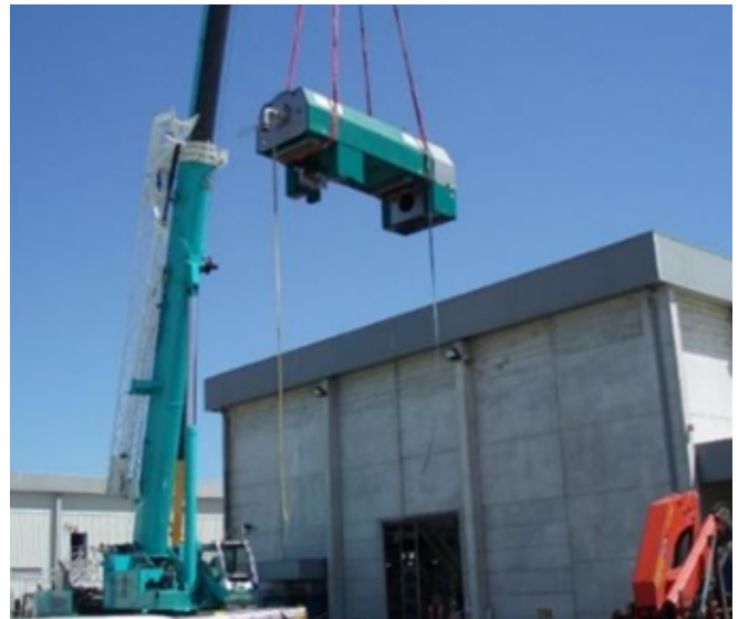
Mangere WWTP, Centrifuge and Conveyor Upgrades, Watercare Services
