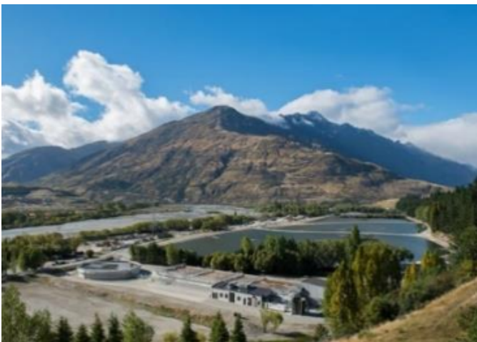
Project Shotover WWTP, Queenstown Lakes District Council
